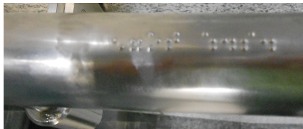
Figure 1: Braille on handrail
